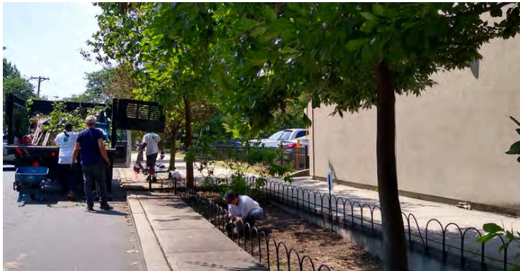
Green Streets crew maintaining a rain garden in Highland Park
